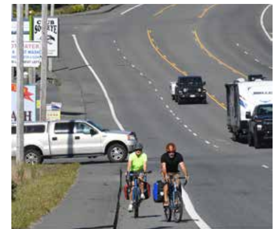
Urban arterial with five lanes for motor vehicle travel and many accesses.
