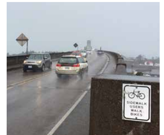
Yaquina Bay Bridge in Newport.
